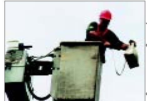
Deploying a bucket evacuation system.
